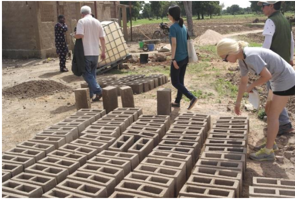
Monitoring the construction of CPAF
